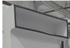
Air conditioning cold air outlet
